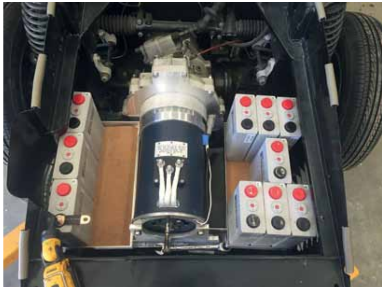
Motor in position with front battery trays fabricated.
