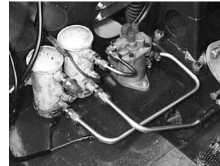
Original Bendix pumps and float chamber. The fuel lines are 10 mm stainless pipe; this also runs to the fuel tank. The bore size of the fuel pipe has been increased to eliminate the chance of fuel starvation because of the tuned engine and large main jets in the carbs.
