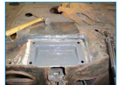
New patch ready to be welded in place.
