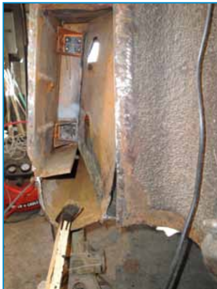
A paint brush on a long stick was used to coat the inside of the rockers.
