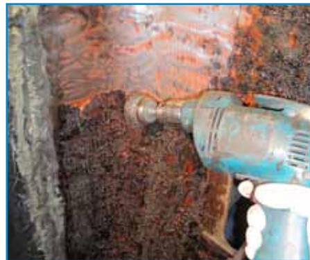
Paint remover and a wire wheel removes undercoating with ease.
